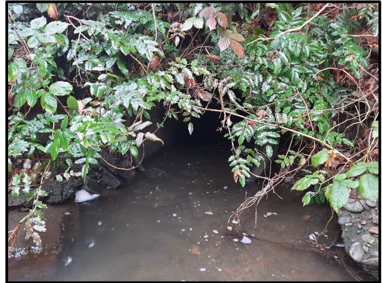
Fever Creek, culvert flowing into the review area
