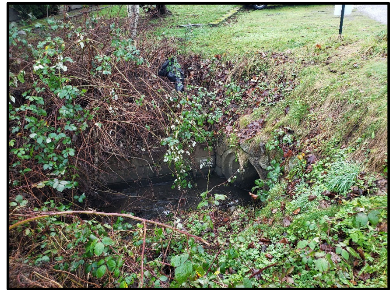
Fever Creek flowing into culvert under Xenia Street (off site)
